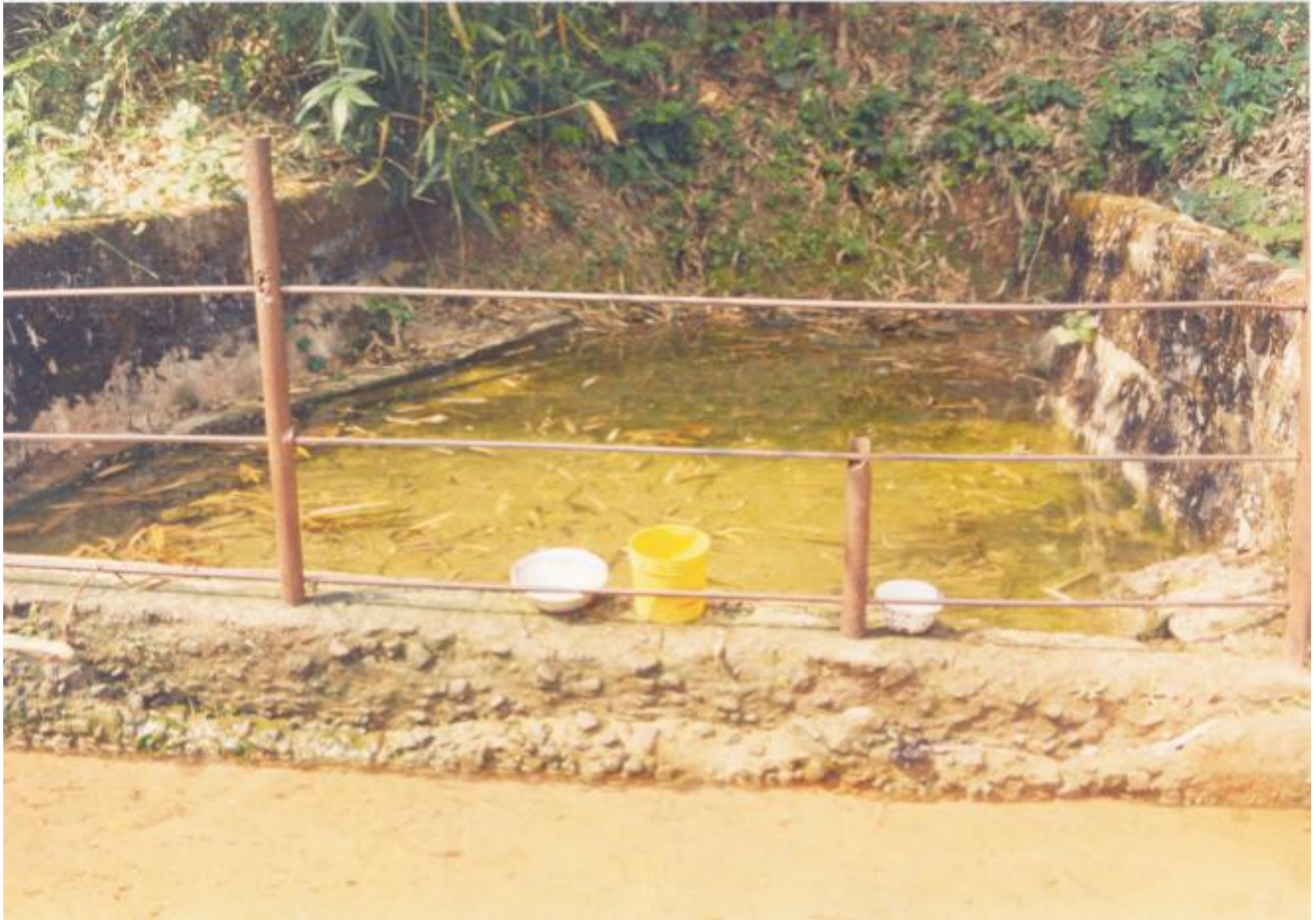
PIC. 1 GROUNDWATER DISCHARGE AT THE BASE OF THE ESCARPMENT
